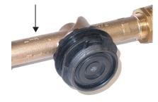
2. When installing the FAM Flow Tube with Plug, be sure to vertically level the Plug for future replacement with FAM Measuring Unit. Turn tap on to release any trapped air in line to the house/apartment. After air is released spot check for leaks around the installation.
