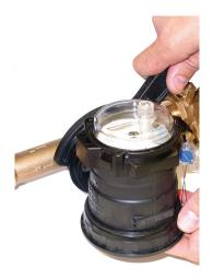
2. After Installing and leveling the meter vertically, check to see if the Measuring unit is level horizontally. Level the Measuring Unit by loosening the locking nut clockwise, adjusting the Measuring Unit and tighten nut counter clockwise.
