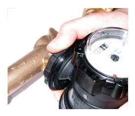
5. Tighten Locking Nut with FAM wrench until snug; do not over tighten. For leveling with level refer to F1 and F2.
